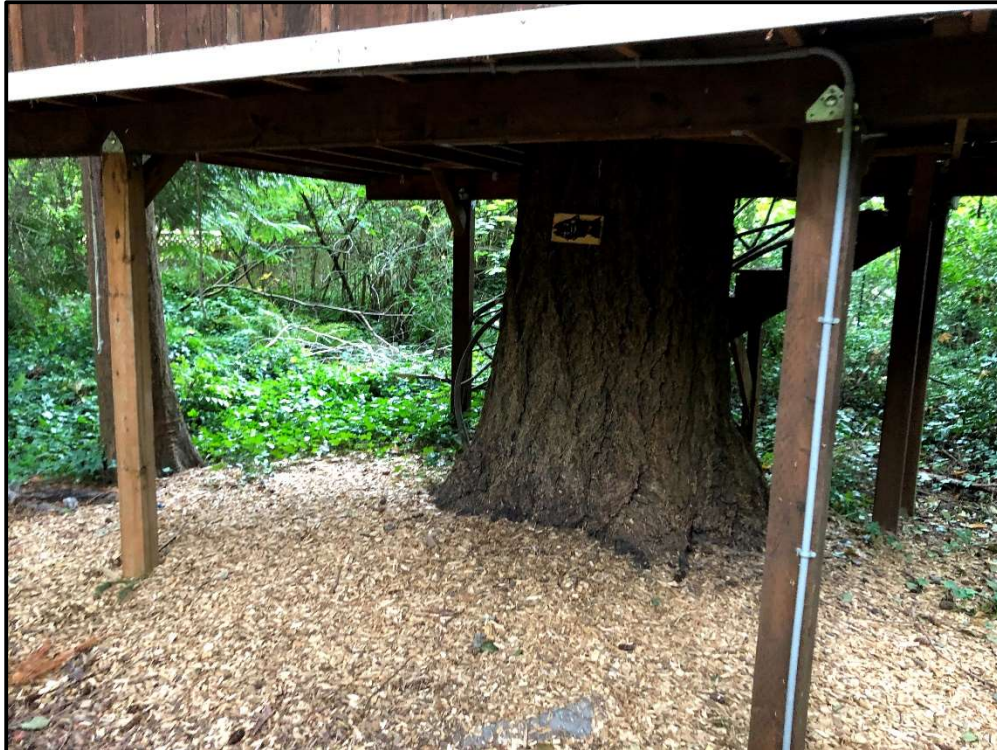
Photo 3. Tree 1806 is not serving as a primary support but is in the center of the treehouse with small attachment hardware. Large diameter surface roots are just below landscape fabric and mulch layer.
