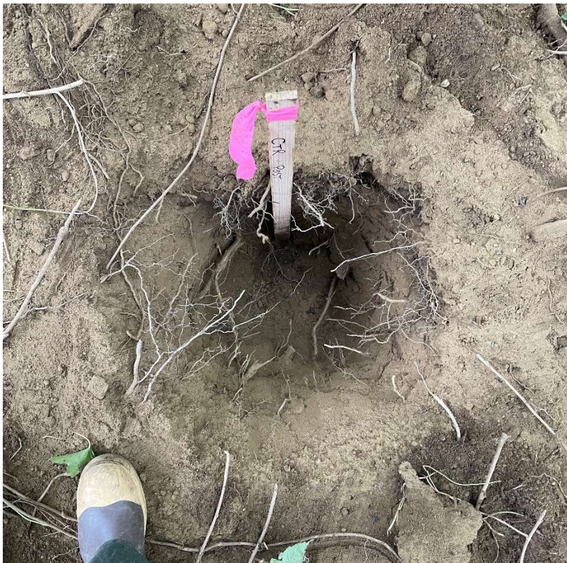
Photo 6. A view of the air excavation at deck footing 2, which is 17 feet to the east of tree 1813. No structural roots were found.
